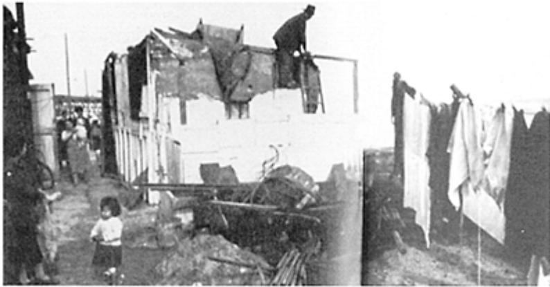
Figure 1.1 Repairs being made to the roof of a shanty dwelling in Poble Nou, circa 1930
