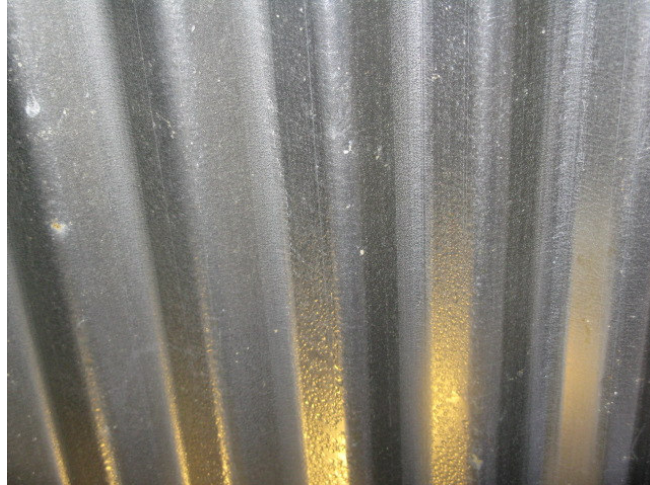
Fig 8: On arrival to Happy Valley, the government provides residents with a housing starter kit, which consists of plastic sheets, corrugated iron and poles (People's Post “No joy as Happy Valley looms large” 13 March 2007). Corrugated iron sweats due to the body heat produced in the overpopulated shelters, which makes the dwellers sick.
