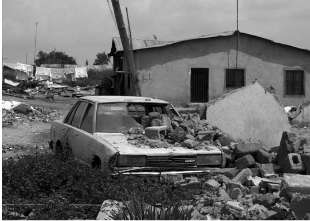
Demolitions in Aleita [Photo: Deanna Fowler, 1 Nov. 2006]
