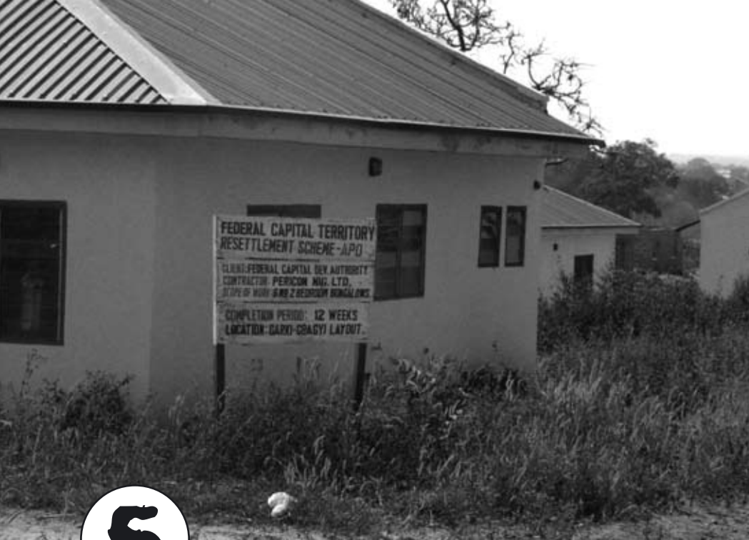
Apo resettlement site construction [Photo: Deanna Fowler, Dec. 2006]
