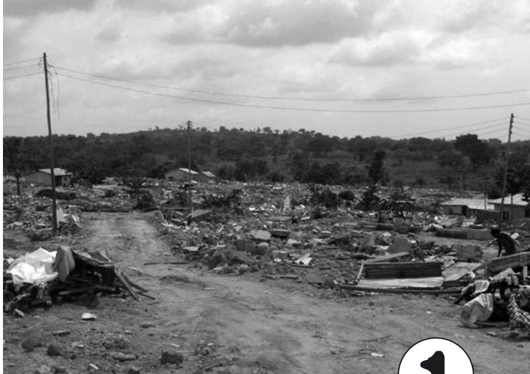
Aftermath of the demolition of Aleita settlement [Photo: Deanna Fowler, 1 Nov. 2006]
