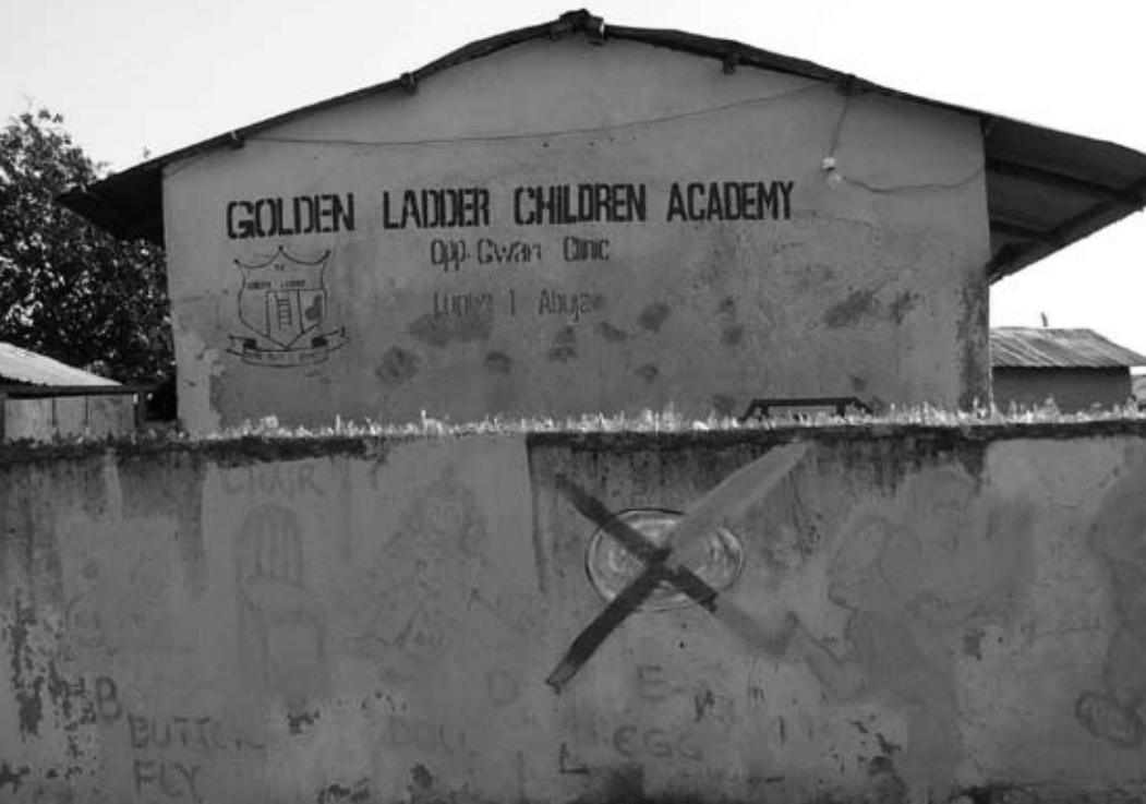
Crèche marked for demolition, Lugbe [Photo: Marie Huchzermeyer, 8 Nov. 2006]
