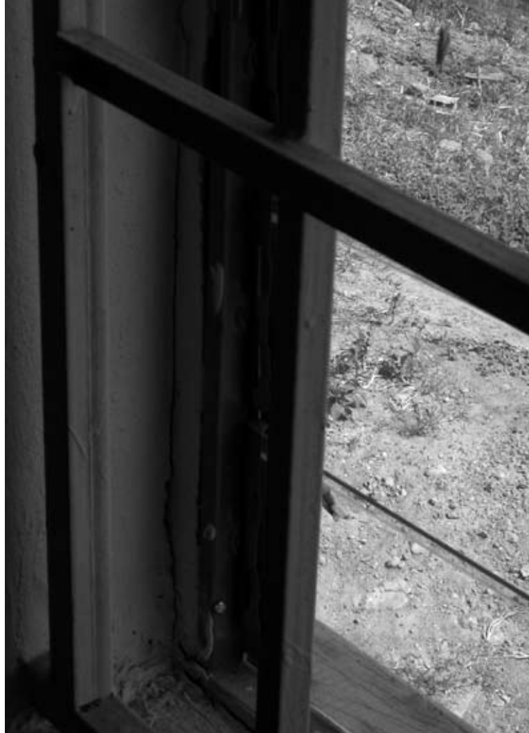
Cracks in new homes at Apo [Photo: Deanna Fowler, Dec. 2007]
