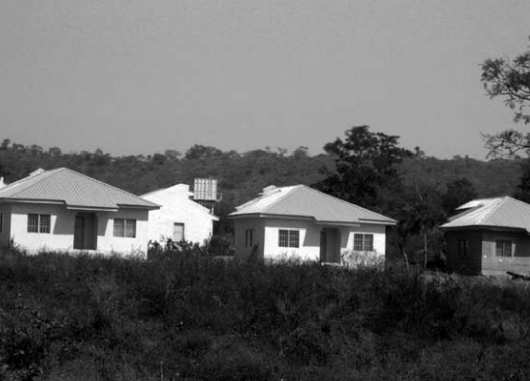
Apo resettlement site: varied quality of construction [Photo: Deanna Fowler, Dec. 2006]
