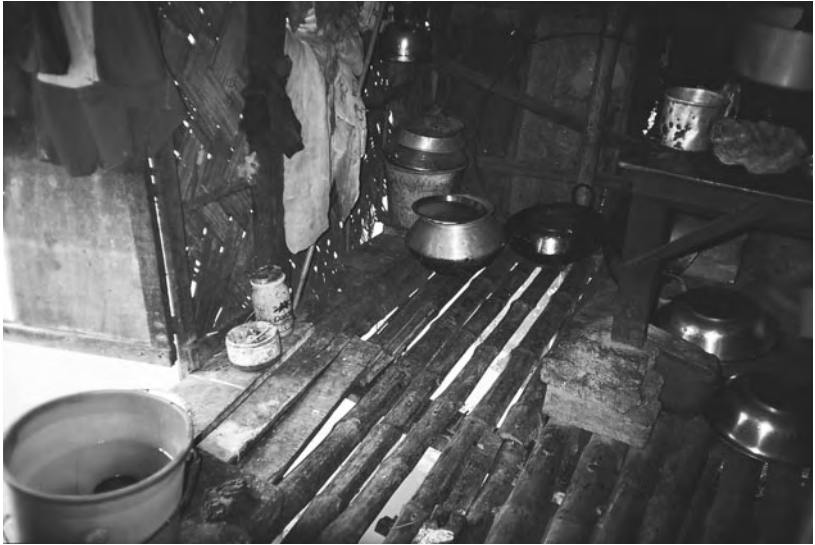
Figure 3.1. The see-through floor of the house on stilts, Jadavpur settlement.
