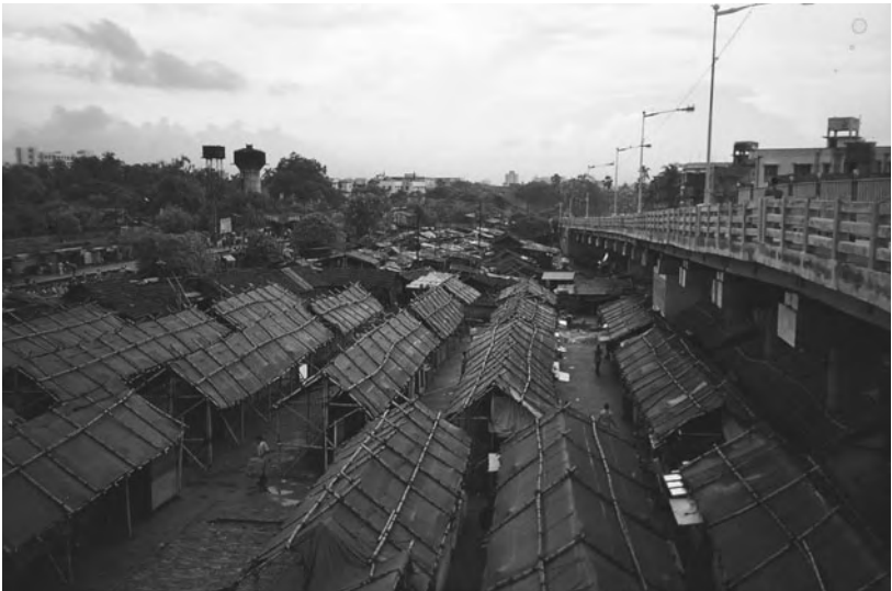
Figure 4.9. Hawker rehabilitation stalls at the Jadavpur station.
