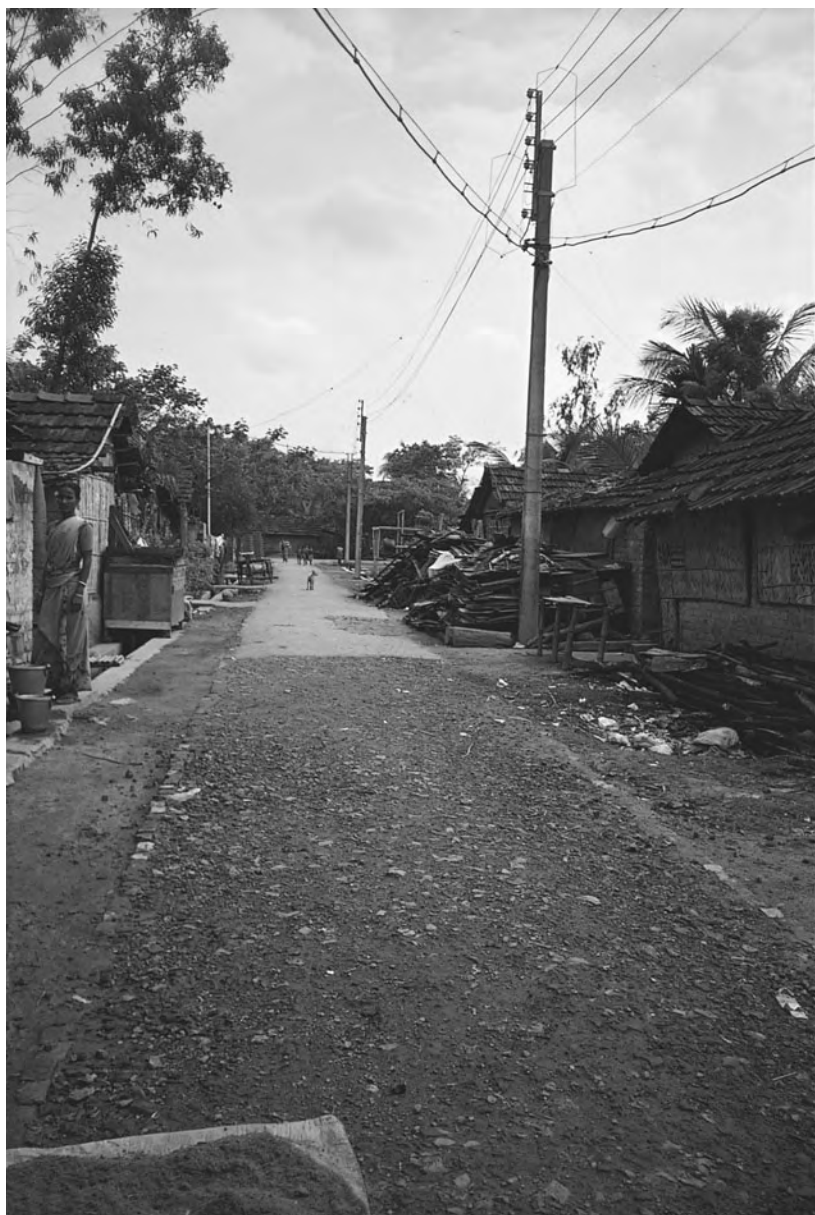
Figure 4.5. Infrastructure: electricity and semifinished roads at the Sahid City colony.
