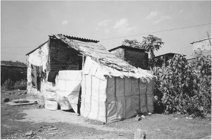
Figure 3.2. Life on the fringes: Swapan and Sumitra's Patuli unit with an extension built with material gathered from construction sites.
