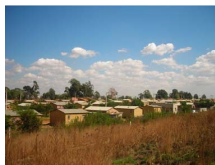
Kingsway RDP housing (established 1989)
