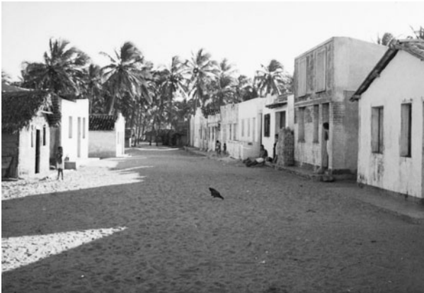
FIGURE P.2 Roof tiles and stucco facades had replaced the thatched palm roofs and packed mud walls of these houses in the center of the settlement.
