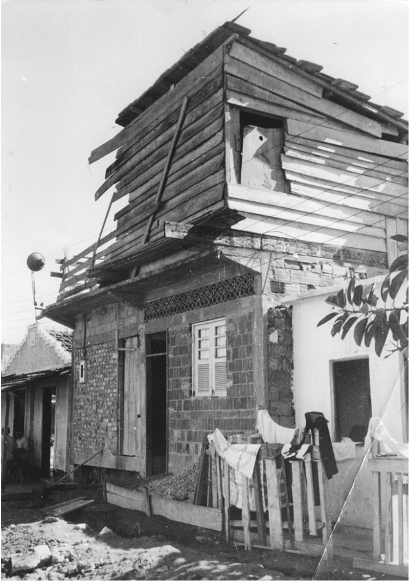
FIGURE 11.2 Barracos in 1968 before CODESCO began upgrading work.
