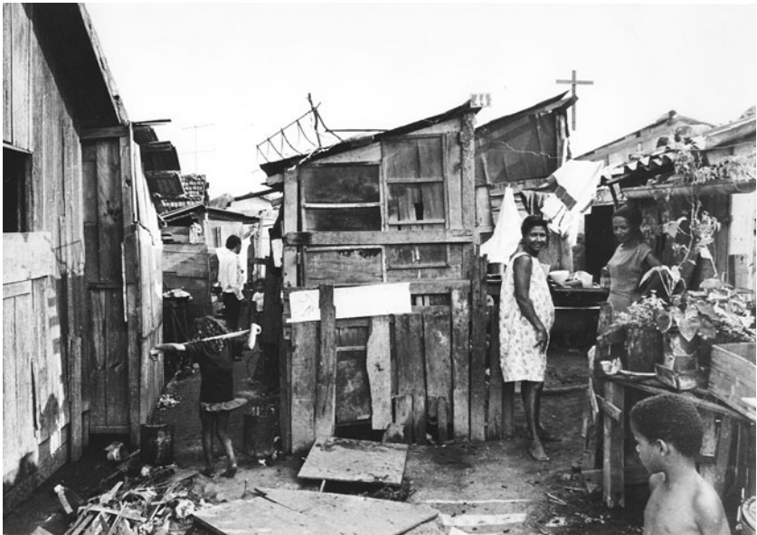
FIGURE 11.1 Barracos in 1968 before CODESCO began upgrading work.
