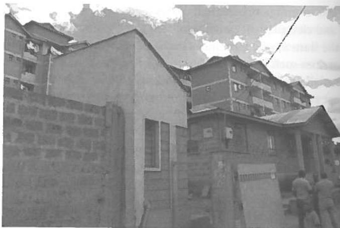
Figure 6.8: The Langata decanting site
