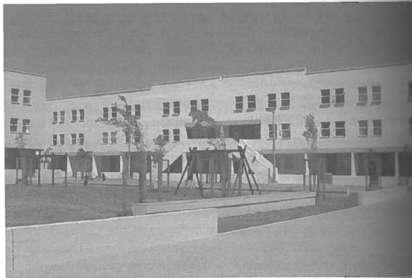
Figure 6.4: Rental housing, Phase One of the N2 Gateway Project
