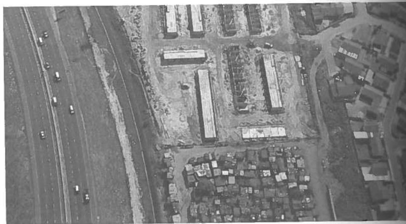
Figure 6.3: Phase One of the N2 Gateway Project under construction in 2005
