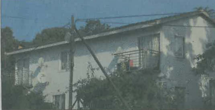
The house in Clare Estate that S'bu Zikode is renting.
